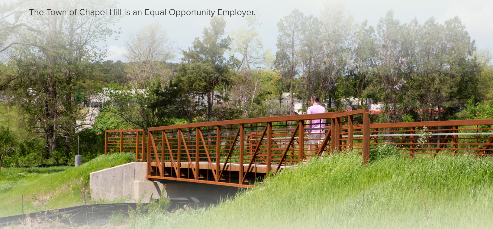
Part of more than 730 acres of public recreation spaces operated and maintained by the Town of Chapel Hill, Booker Creek Basin Park offers a 10' wide paved trail through open meadow and wooded floodplain.
