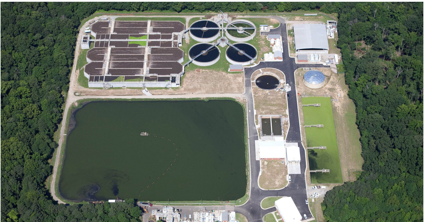
Aerial view of Triangle Wastewater Treatment Plant
